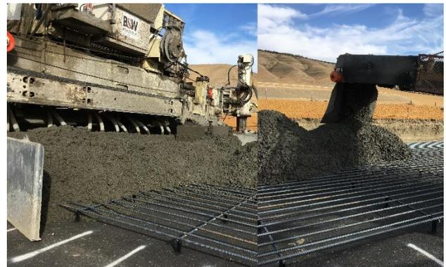
Figure 2. Concrete Dumped Directly in Front of the Paver Using Belt Placer
