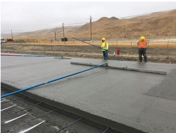
Figure 3. Typical Hand Finishing Procedures
