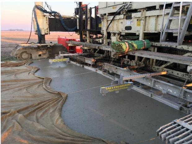
Figure 1. RTP Installed Directly at the Rear of the Paver
