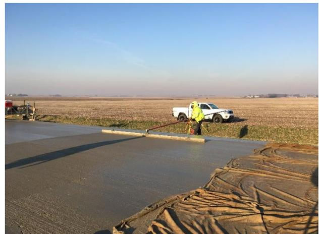
Figure 2. Typical Finishing With a Straightedge
