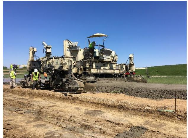
Figure 4. Concrete Spread Ahead of the Paver
