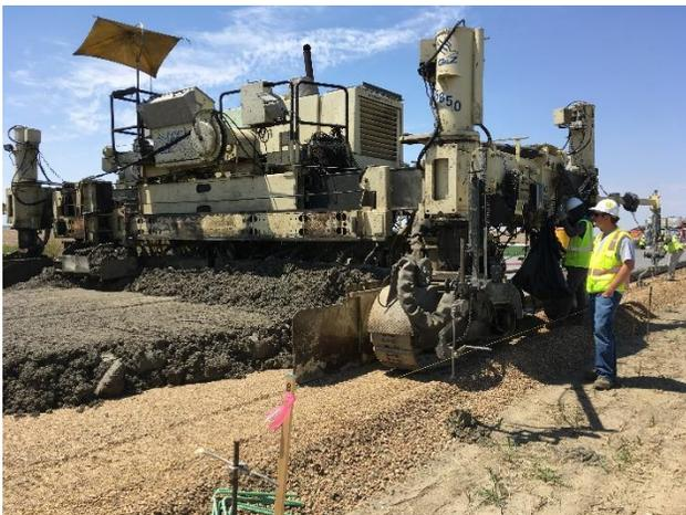
Figure 5. Stable and Trimmed Paver Track Line
