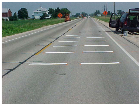
Figure 7-9. Temporary Rumble Strip (Horowitz and Notbohm 2002)
