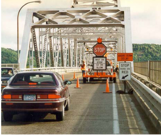
Figure 4-2. AUTOFLAGGER (Mn/DOT 2000)
