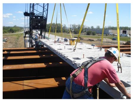
Figure 2.5. Placing precast deck panel on girders
