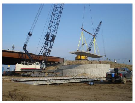
Figure 4.5. Deck panel being lifted into place
