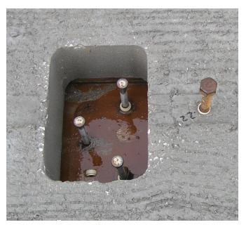
Figure 2.8. Shear stud pocket and studs
