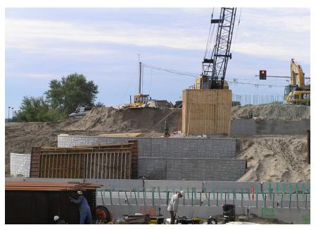
Figure 2.1. Construction of south abutment and terrace walls
