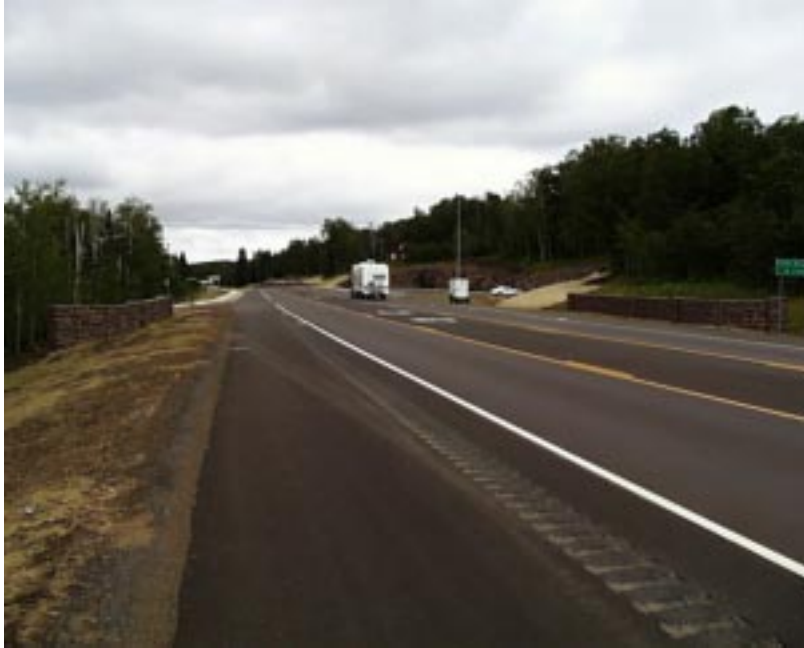
Figure 4.15 New Pavement and Added Two-Way Left-Turn Lane—Schroeder
