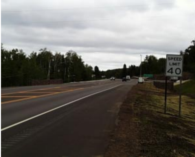
Figure 4.14 Trailer’s Position with Respect to the Gates and Speed Limit Sign—Schroeder
