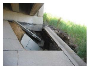
Failure of concrete slope protection due to erosion
