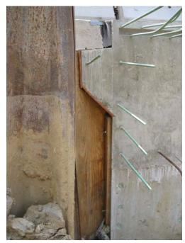
Inclined paving notch observed during construction of a new bridge
