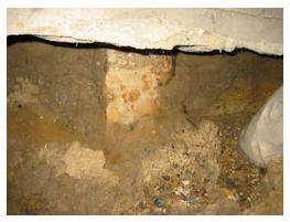
Exposed H-pile caused by soil erosion under the abutment
