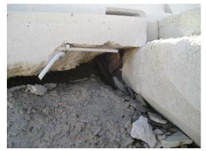
A 9-inch void under the approach slab and spalling of concrete from the paving notch and the approach slab
