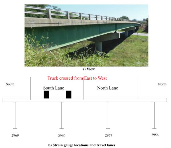
Figure 3.7 Long-span steel girder Bridge 600770 strain gauge locations
