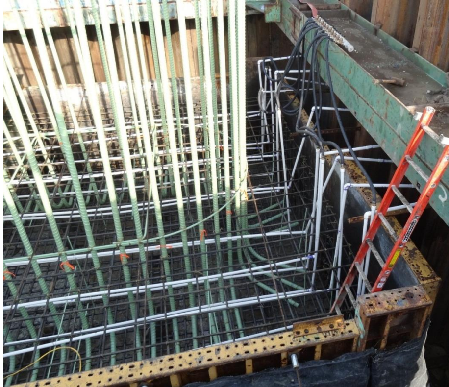
Figure 3.20. Installed PVC piping on US 34 Bridge footing
