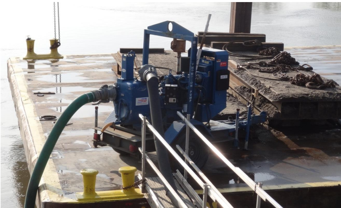
Figure 3.15. US 34 Bridge cooling pipe system water supply pump
