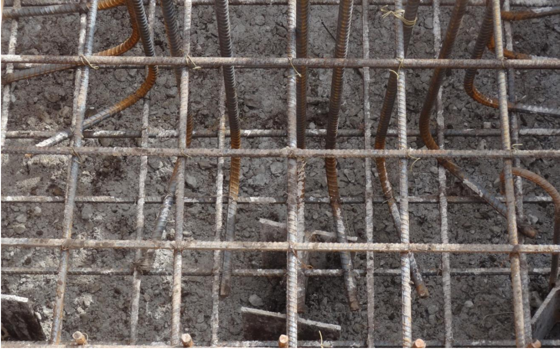
Figure 3.2. Crushed rock subbase with steel bearing pile
