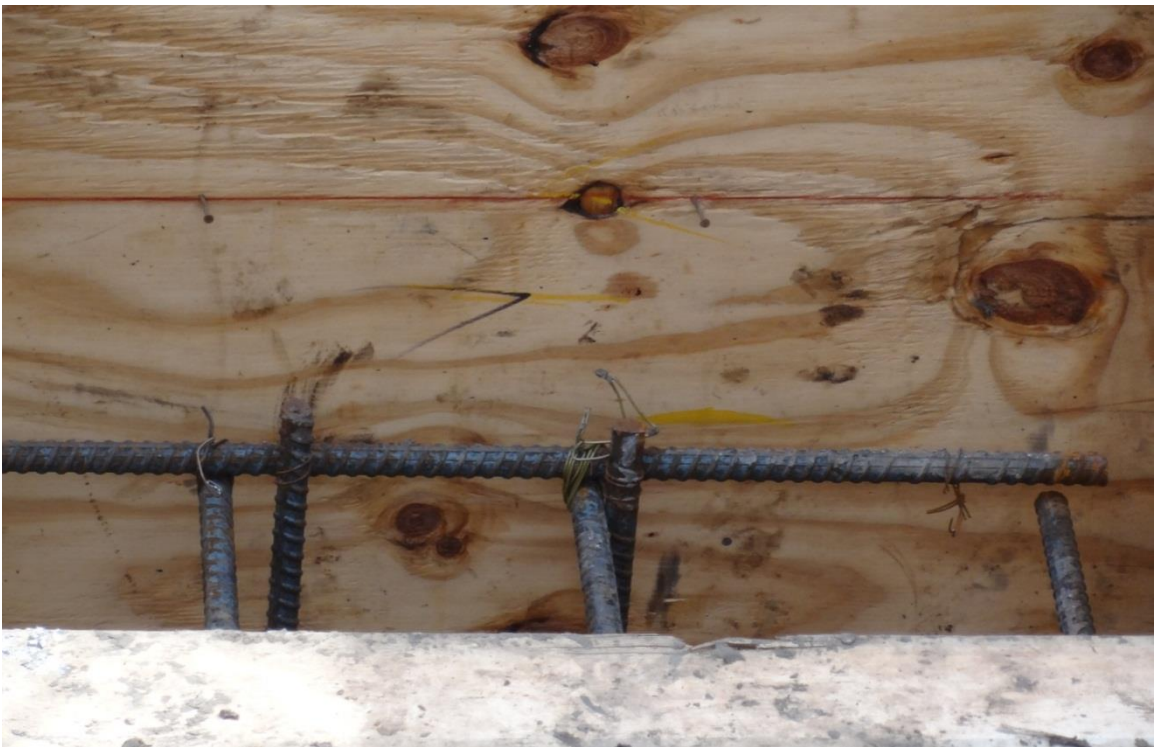
Figure 3.23. Typical rebar cover for mass concrete footing
