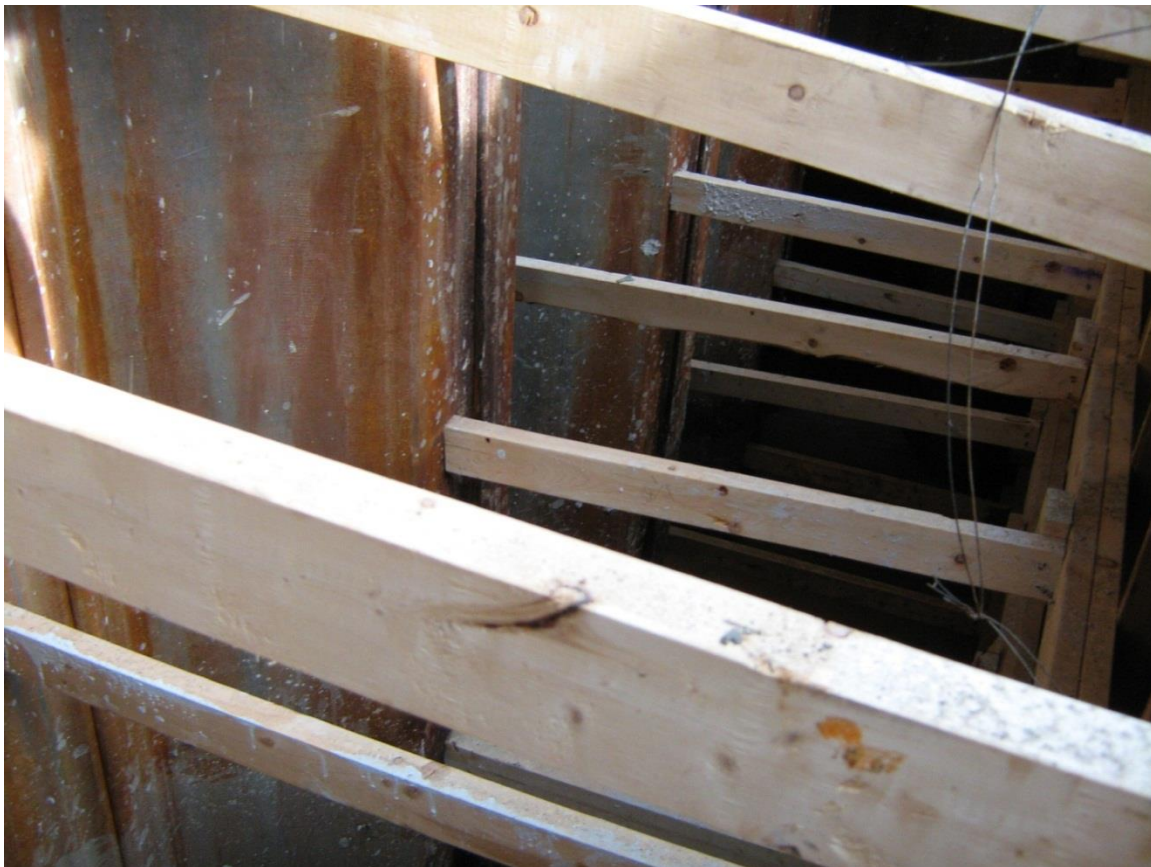
Figure 3.11. WB I-80 Bridge wood-formed footing shoring
