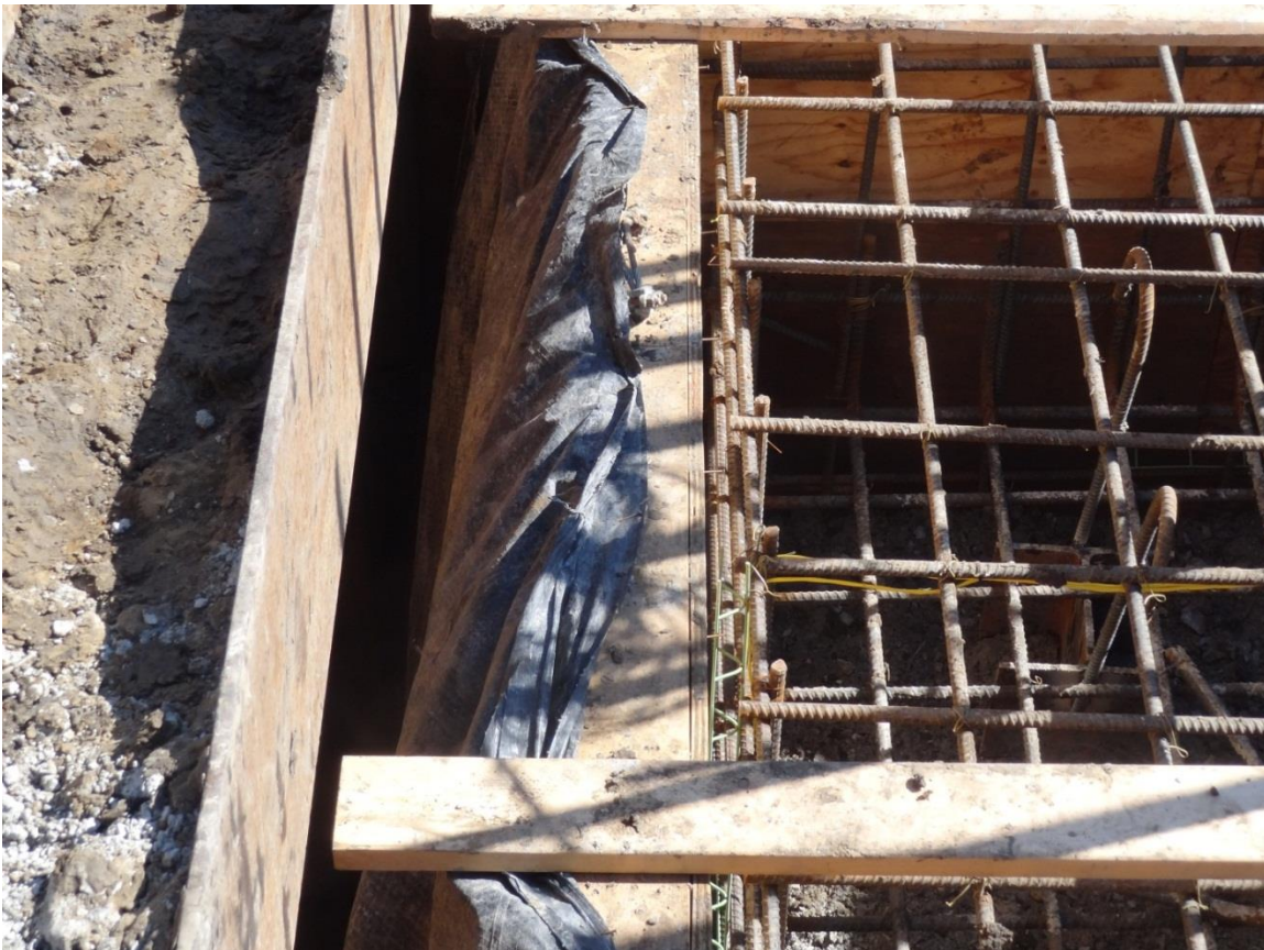
Figure 3.10. Insulation attached to wood-formed footings
