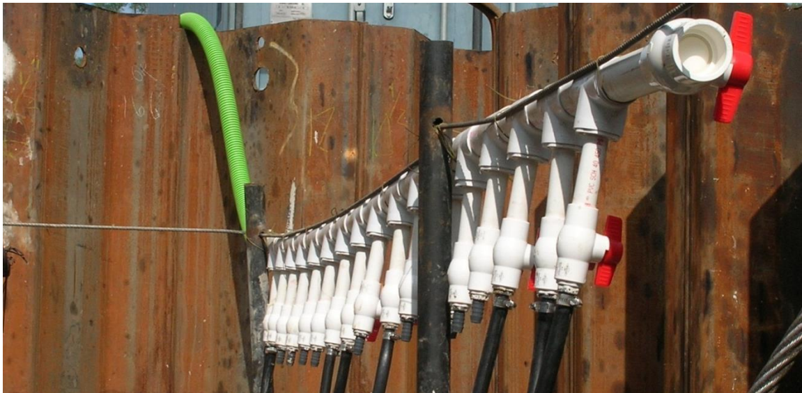
Figure 3.17. WB I-80 Bridge cooling pipe system manifold
