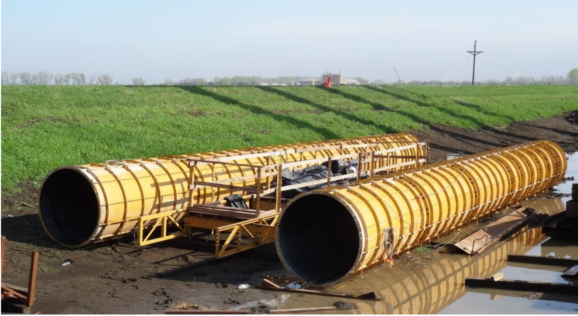
Figure 3.5. US 34 Missouri River Bridge column formwork
