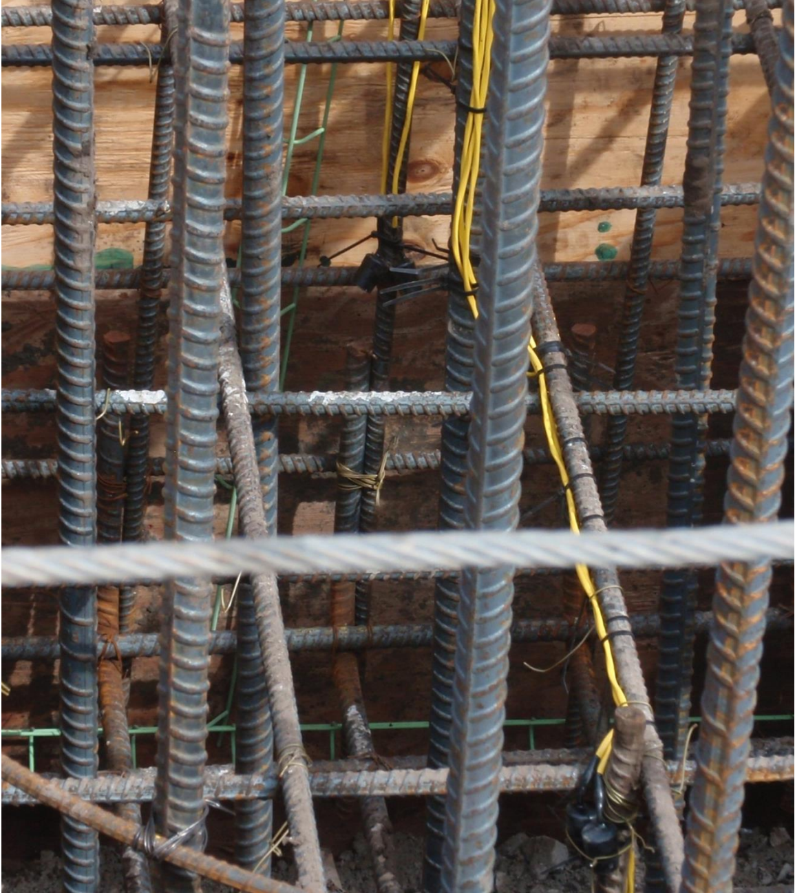
Figure A.5. Typical side surface and center sensor layout
