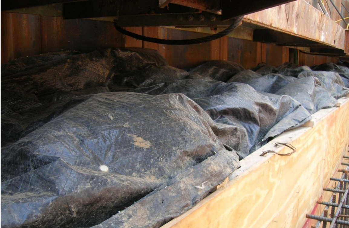
Figure 3.12. Shored formwork insulating blanket
