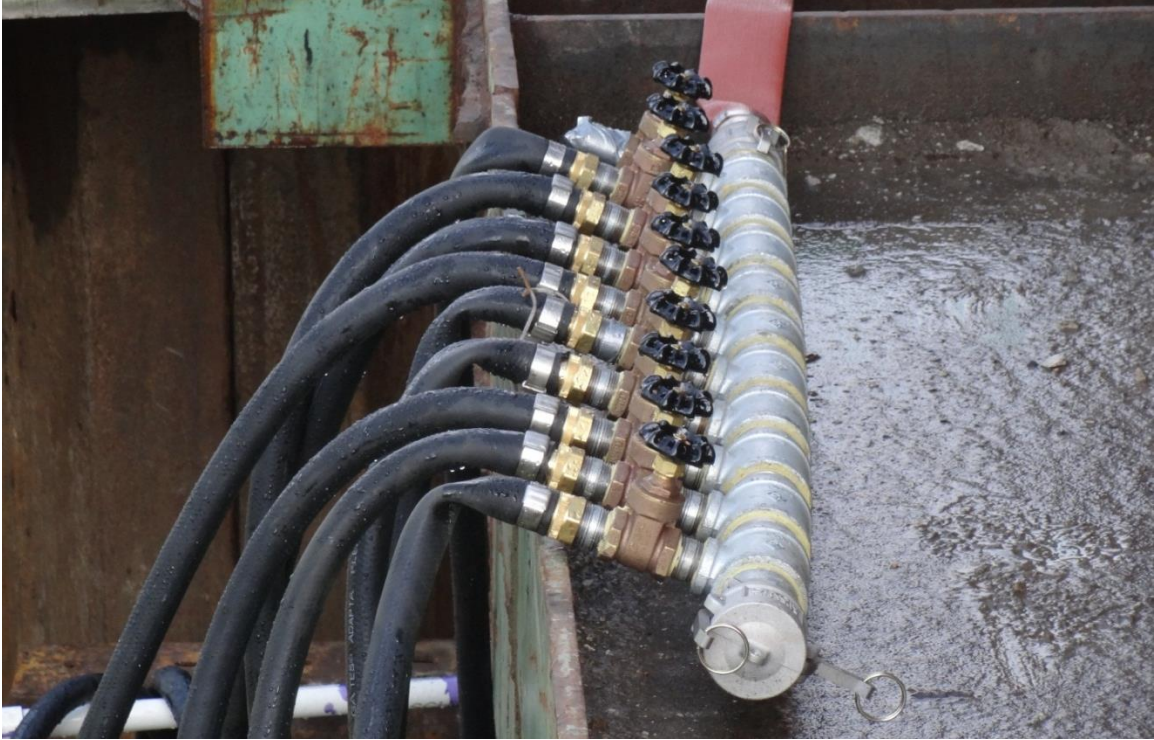
Figure 3.18. US 34 Bridge cooling pipe system manifold
