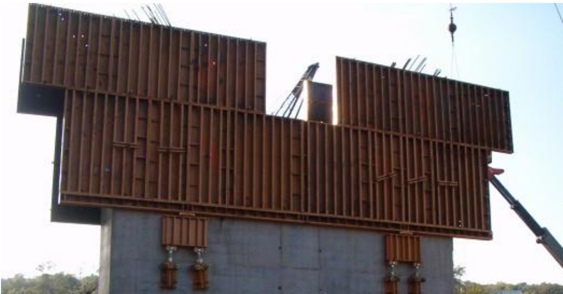
Figure 3.4. WB I-80 Missouri River Bridge column formwork
