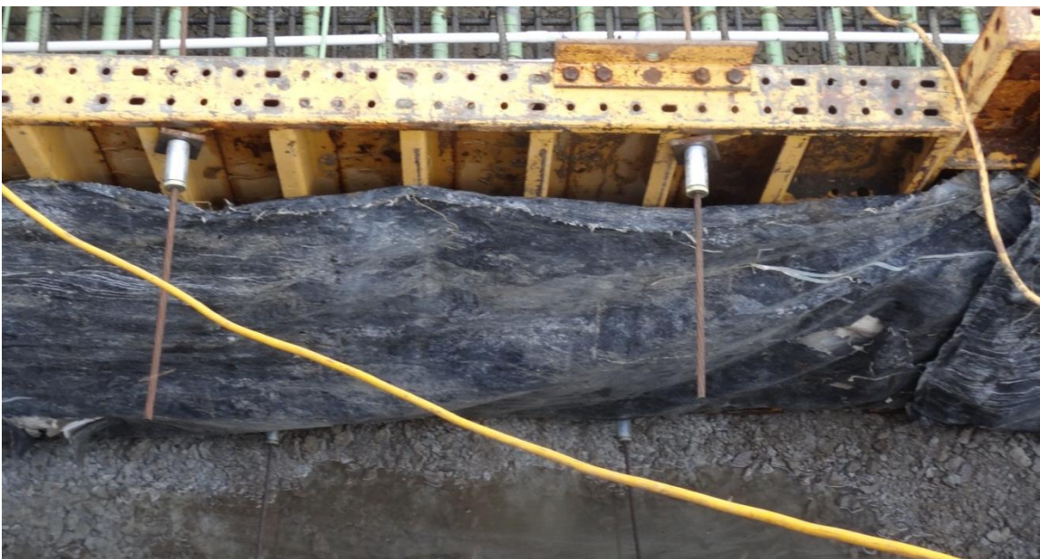
Figure 3.14. Steel formed footing with insulating blanket
