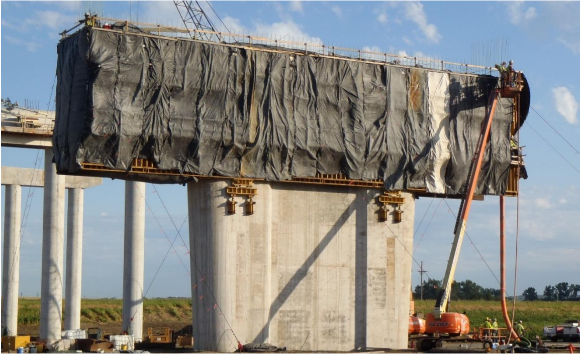
Figure 3.13. Elevated placement with insulating blankets wrapped around the catwalks
