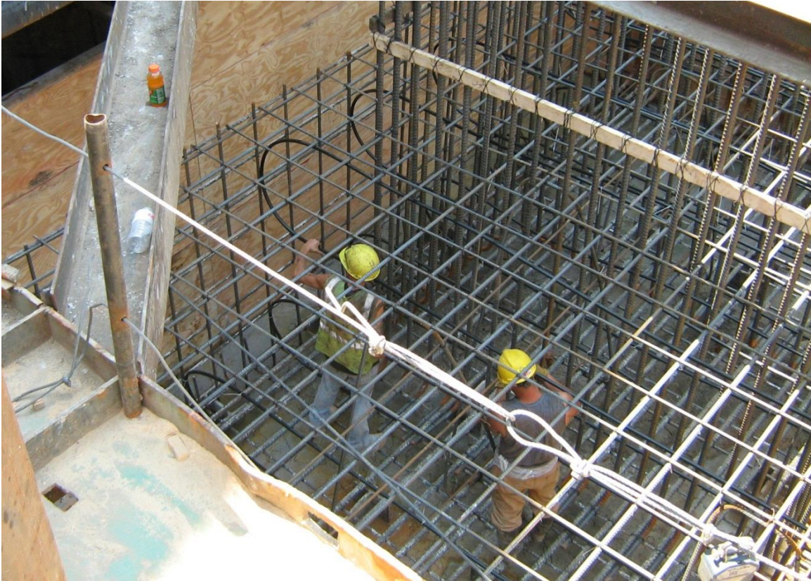
Figure 3.19. PEX cooling pipes being installed on a WB I-80 bridge footing (Iowa DOT)
