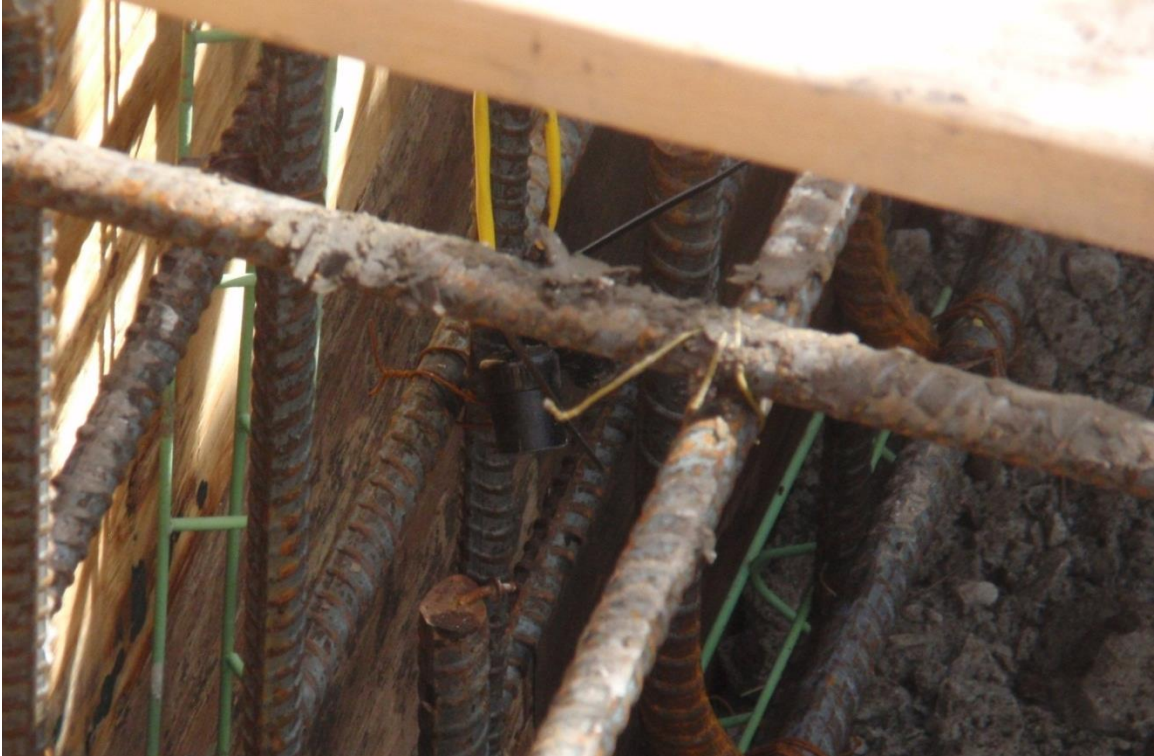
Figure 3.22. Distance between formwork and outermost rebar/thermal sensor location
