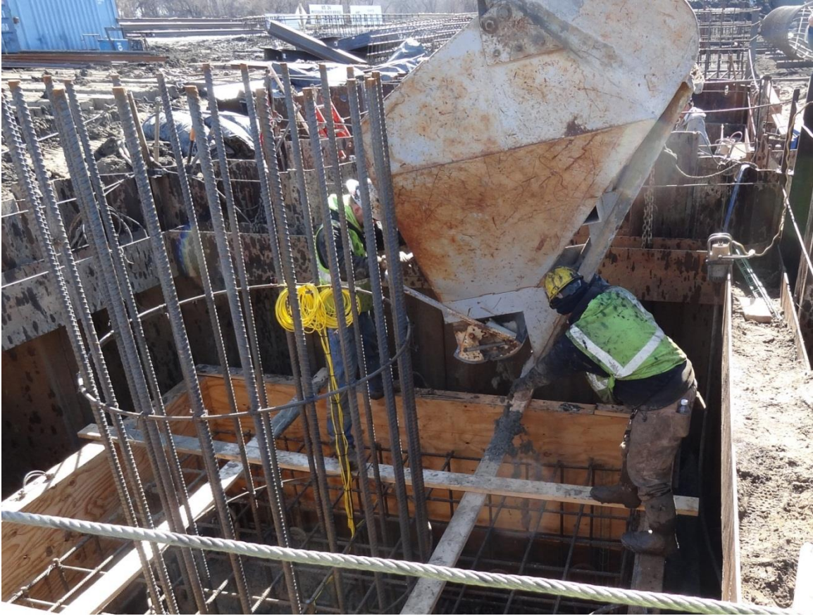
Figure 3.8. US 34 Bridge Pier 2 footing concrete placement
