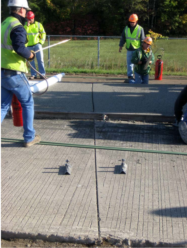
Figure 72. Jointing on fresh pavement
