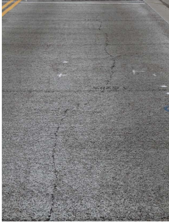
Figure 68. Longitudinal crack from heavy vehicles or loading repetitions
