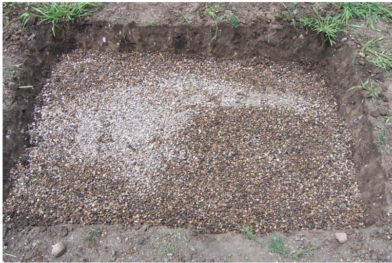
Figure 37. Aggregate base at test location
