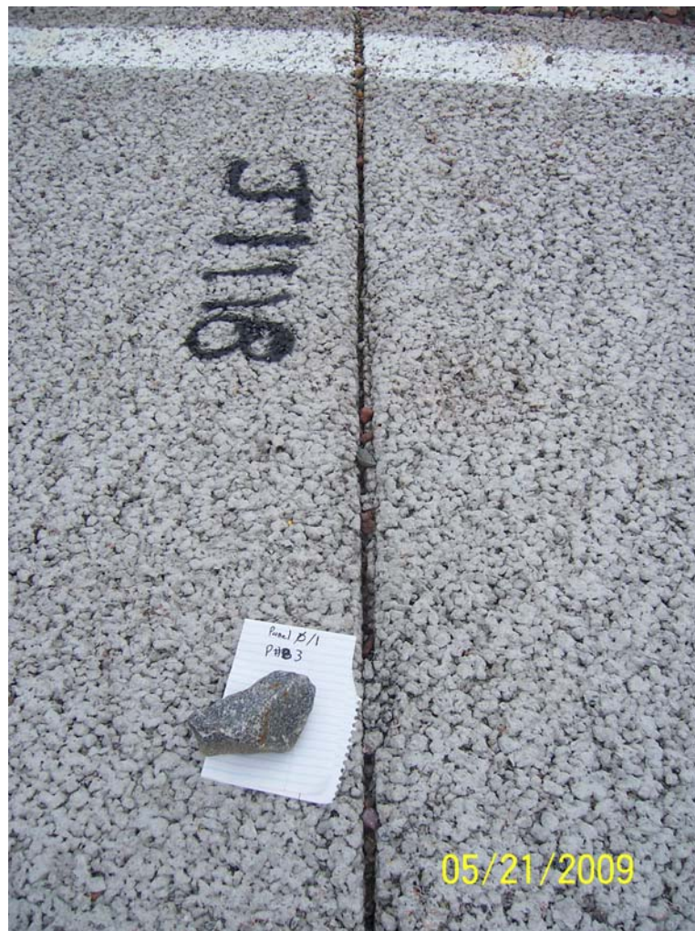
Figure 70. Example of double-jointing
