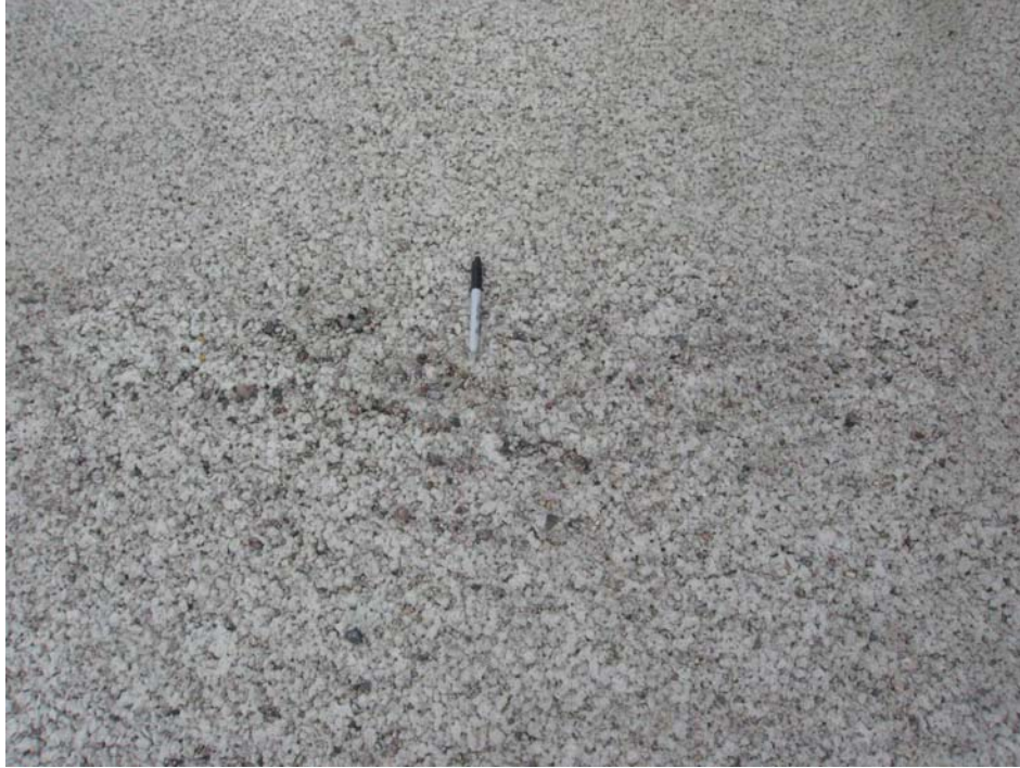
Figure 66. Stretch mark example
