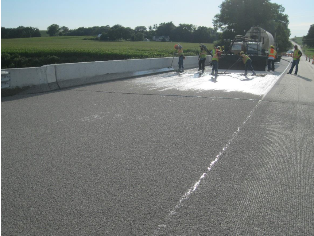
Figure 45. Flint chips spread on the Keg Creek deck
