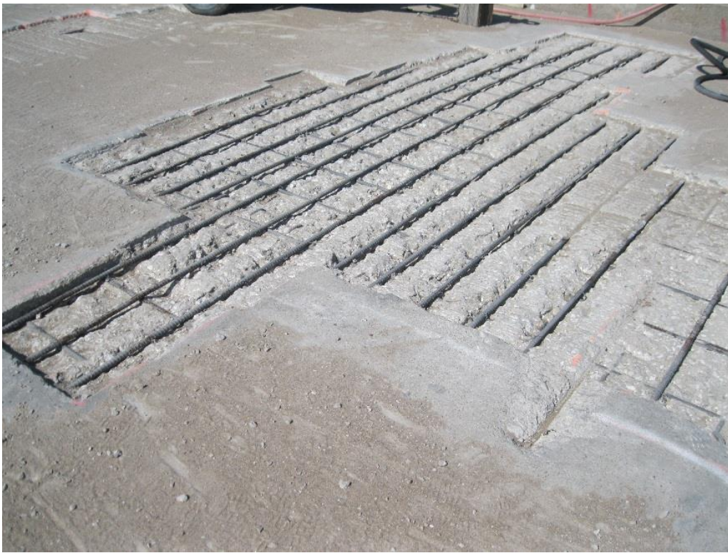
Figure 17. Top reinforcing steel bar mat on Johnson County bridge
