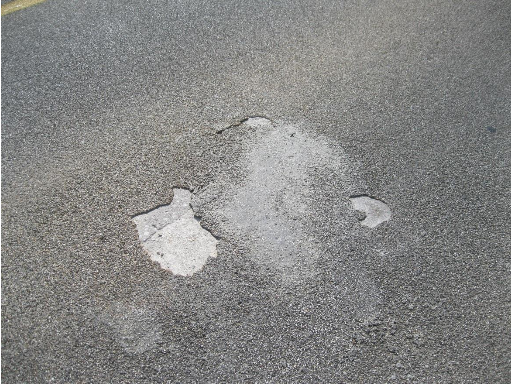
Figure 66. Close-up of delaminated area on Johnson County bridge deck
