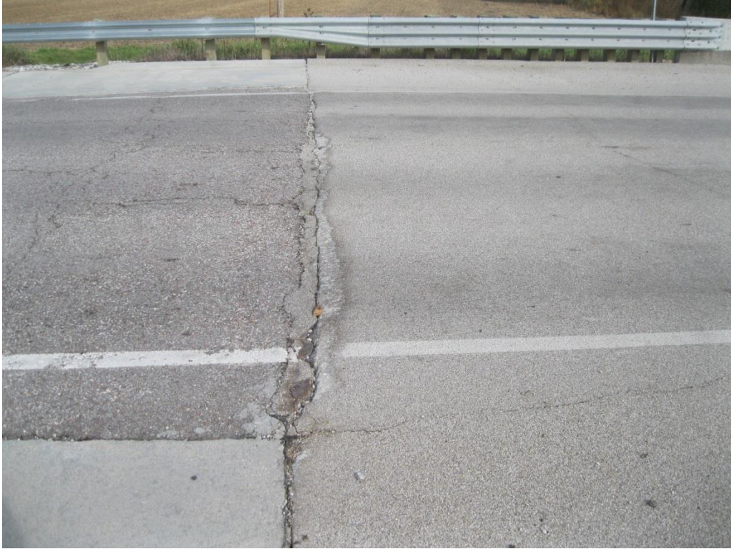
Figure 75. Keg Creek scuffing at approach slab entrance
