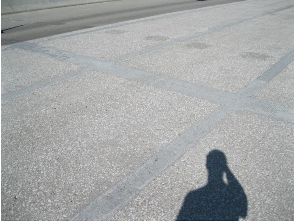
Figure 37. Keg Creek UHPC deck closure pours
