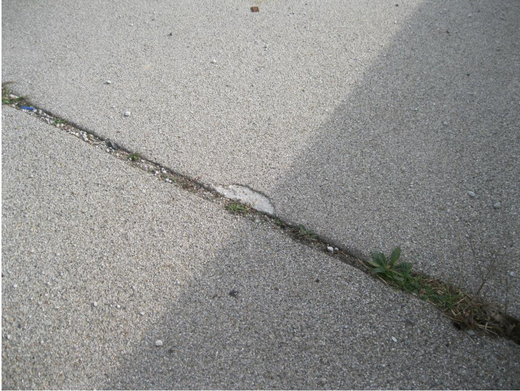
Figure 76. Keg Creek small delamination at end of deck
