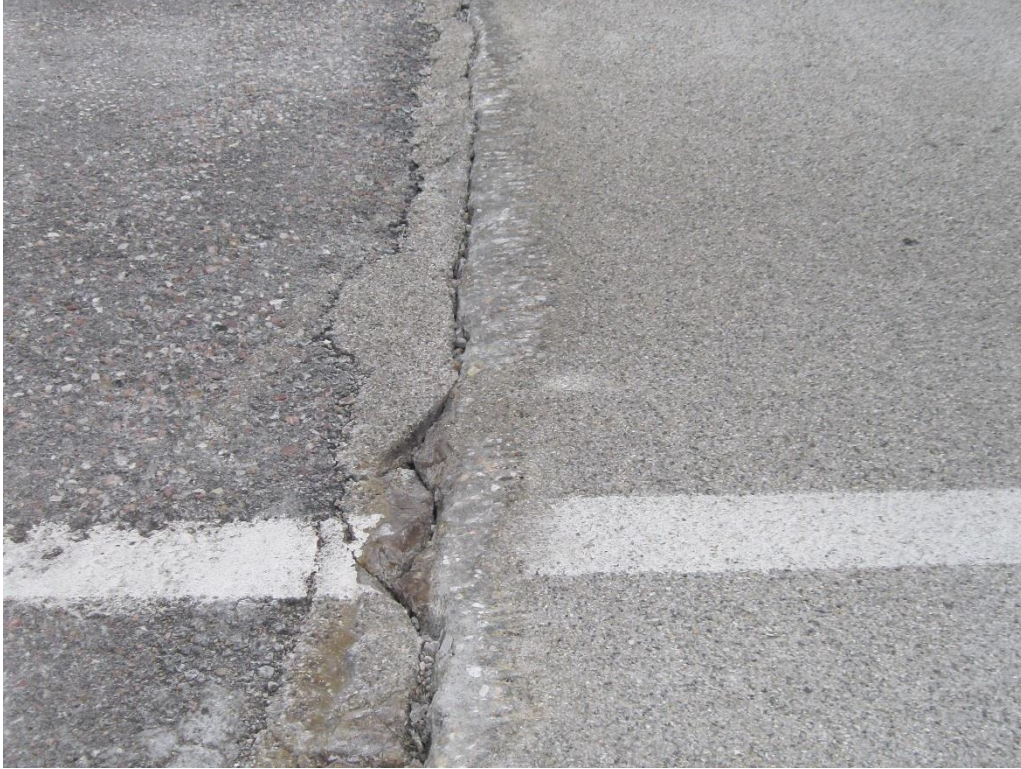
Figure 71. Keg Creek scuffing from plow at bridge entrance
