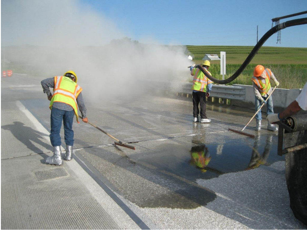
Figure 44. Blowing flint chips into polymer on the Keg Creek deck
