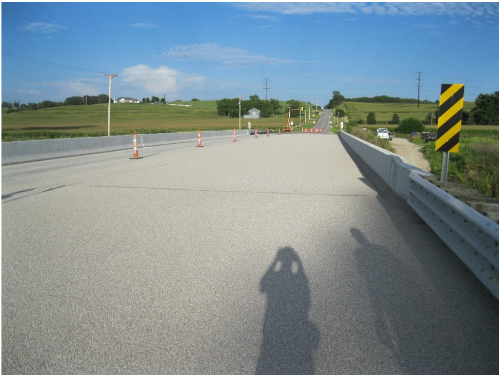
Figure 46. Finished flint chip application on the Keg Creek deck
