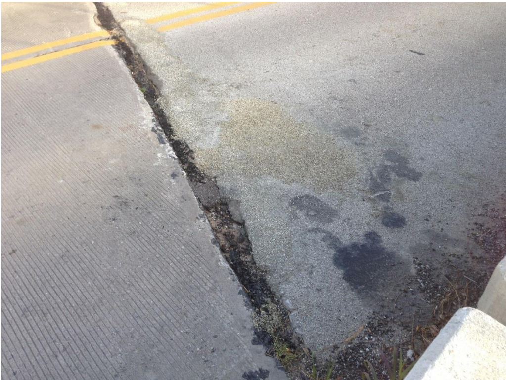
Figure 54. Johnson County epoxy polymer repair at north end of bridge
