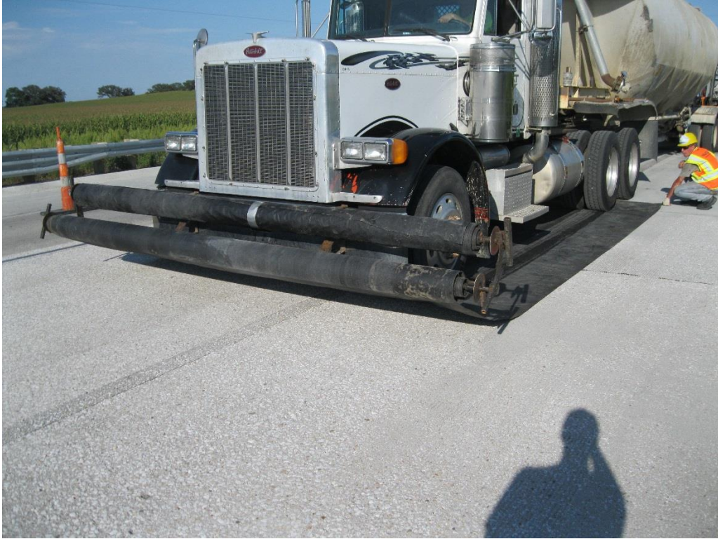
Figure 41. Keg Creek deck protection
