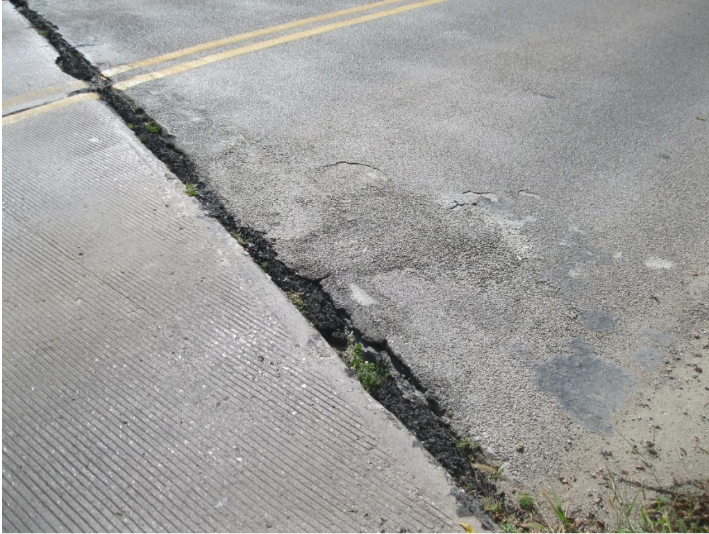
Figure 64. Johnson County expansion joint at north end of bridge
