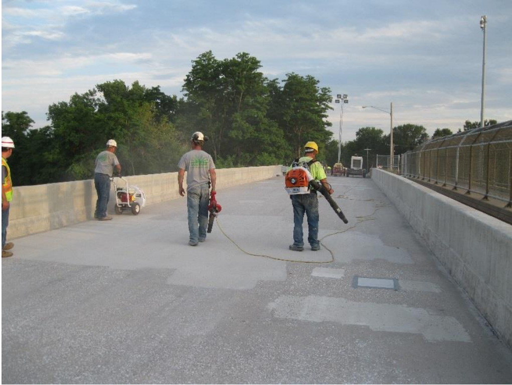
Figure 22. Johnson County deck cleaning
