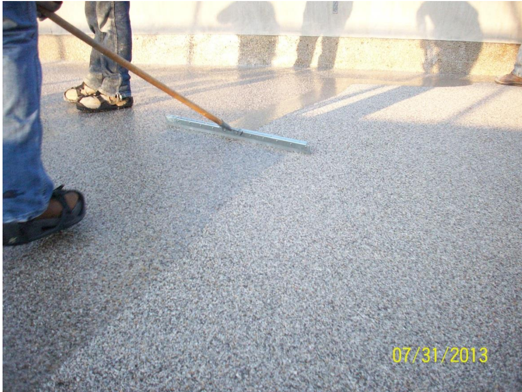
Figure 34. Second layer of polymer application on Johnson County deck
