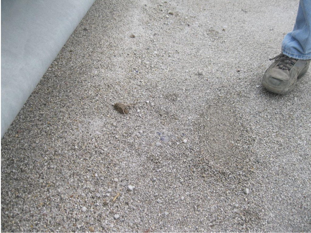
Figure 68. Keg Creek collection of cast aggregate at curb line (1 of 2)
