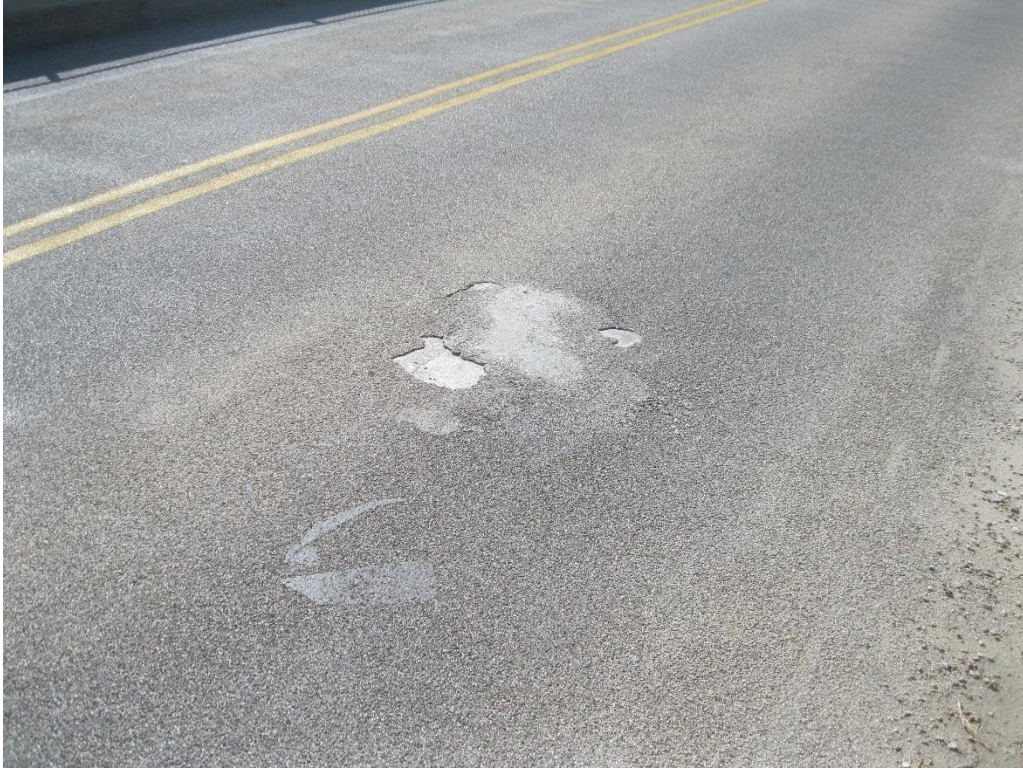
Figure 65. Johnson County delaminated area north of the center pier in the southbound lane
