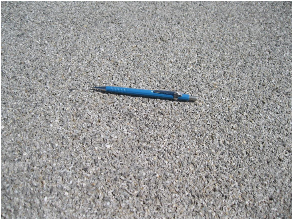
Figure 81. Keg Creek surface roughness outside of wheel line smoothing
