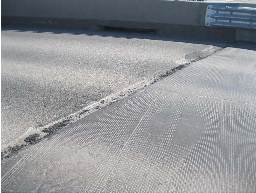
Figure 50. Johnson County delamination at south end of bridge (1 of 2)
