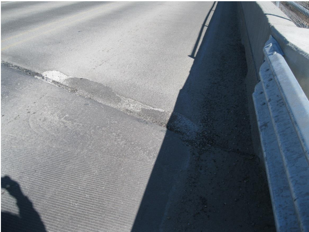
Figure 51. Johnson County delamination at south end of bridge (2 of 2)
