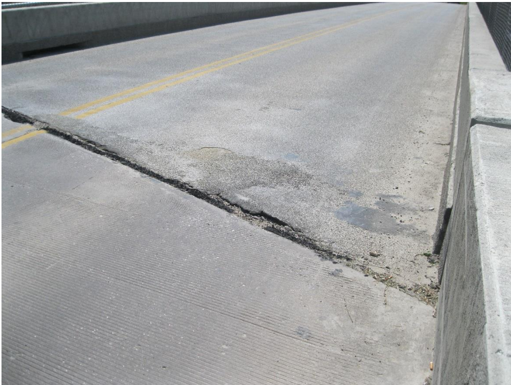
Figure 59. Johnson County epoxy polymer repair at north end of bridge (2 of 2)
