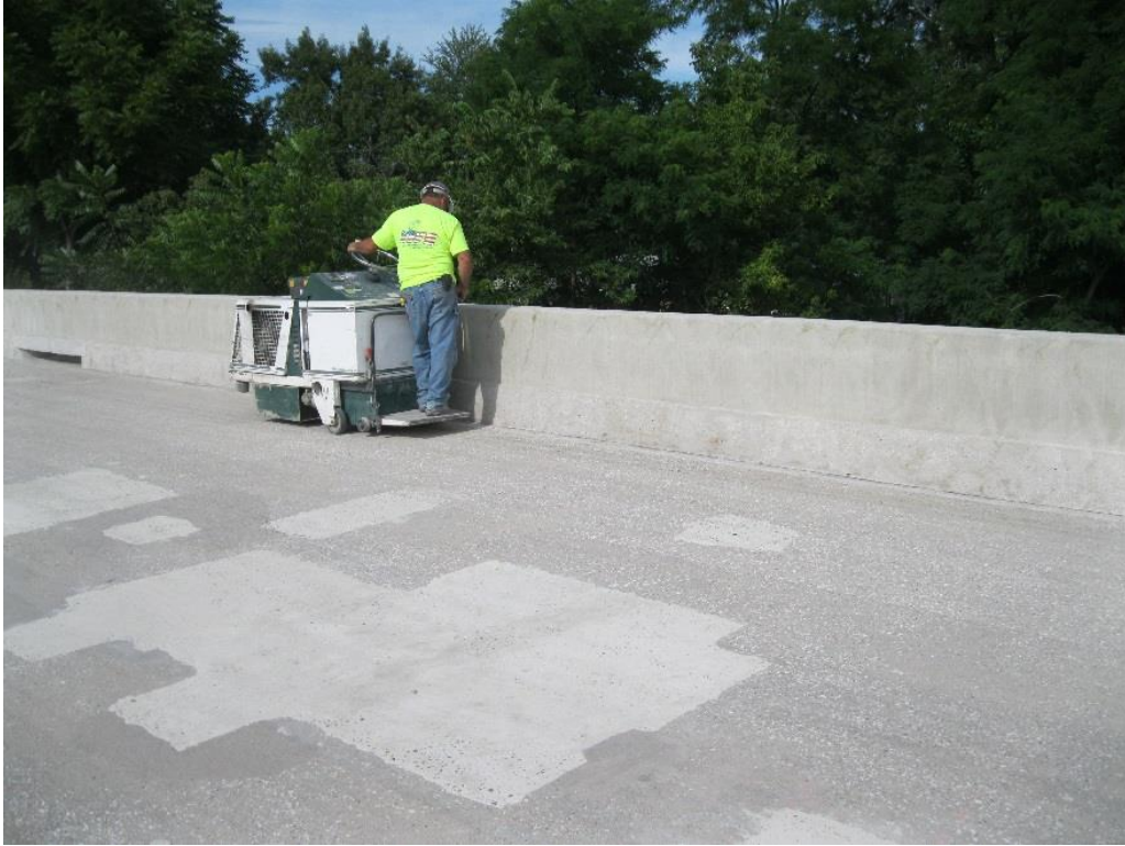
Figure 20. Shot blasting Johnson County bridge deck
