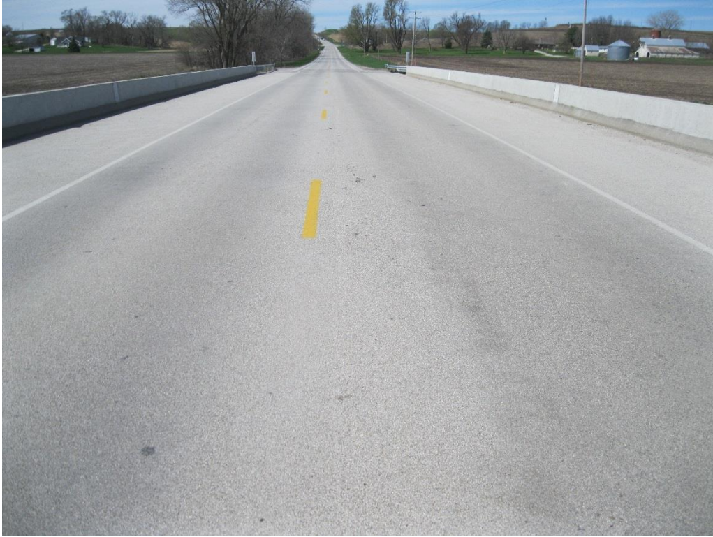
Figure 79. Keg Creek wheel line smoothing
