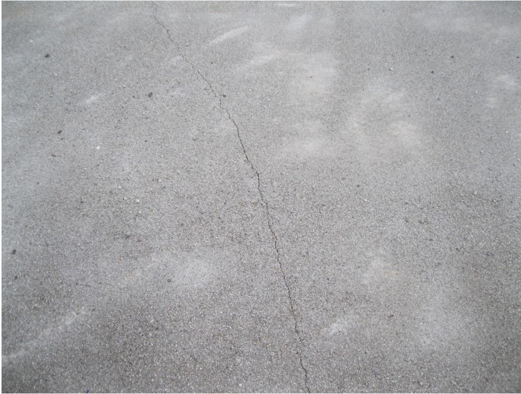
Figure 70. Keg Creek reflective cracking in approach slabs
