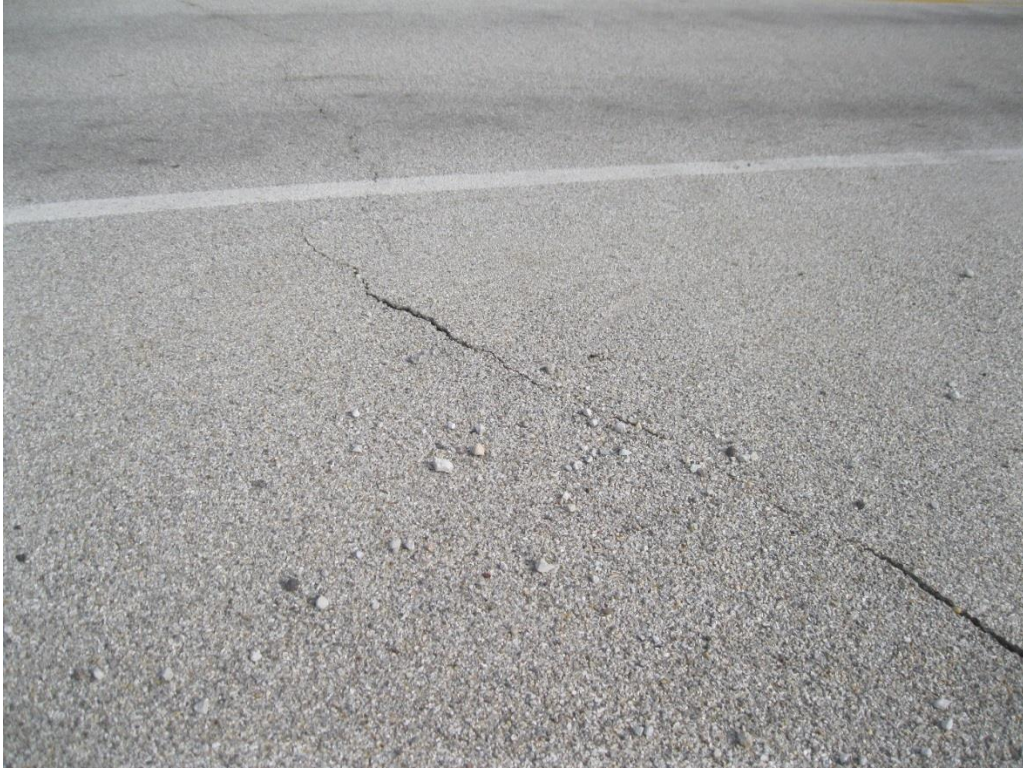
Figure 74. Keg Creek reflective cracking in approach slab
