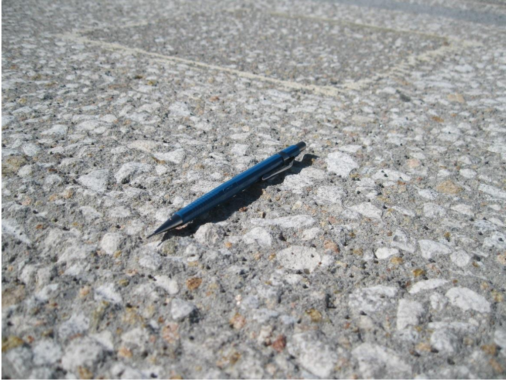
Figure 40. Keg Creek surface roughness
