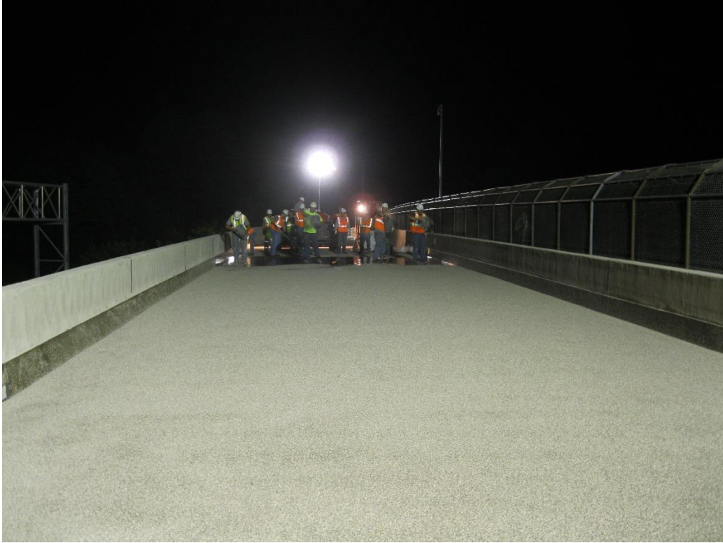
Figure 30. First layer progress on Johnson County bridge deck
