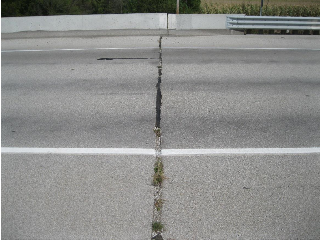
Figure 84. Keg Creek expansion joint
