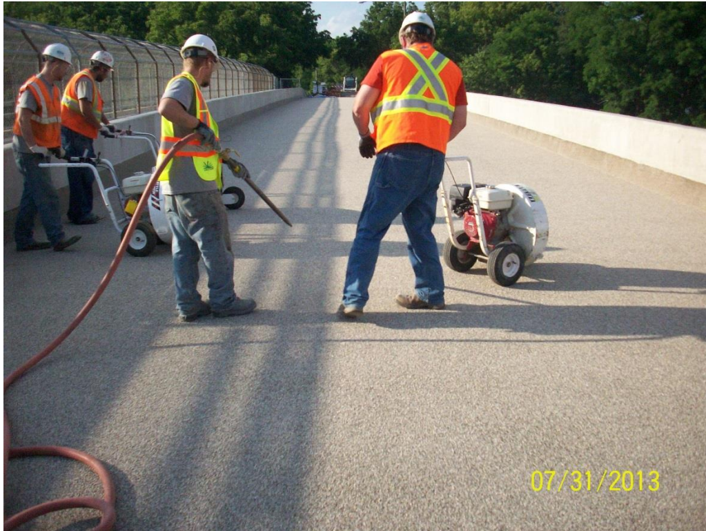
Figure 32. Johnson County deck preparation prior to second layer application
