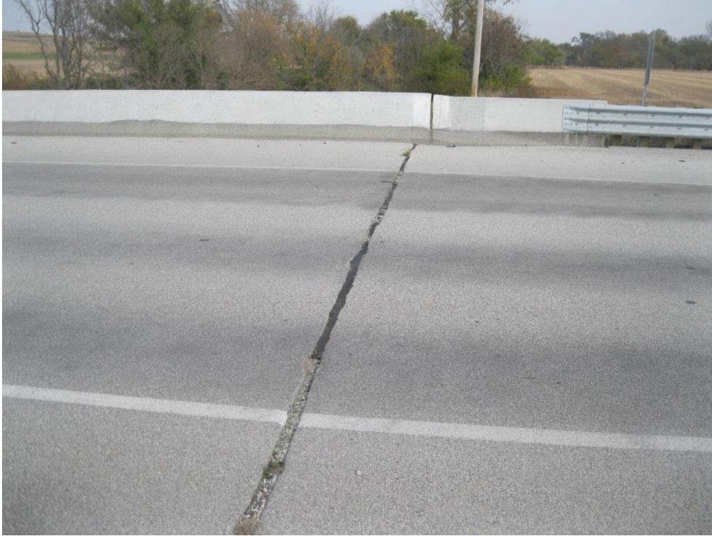
Figure 73. Keg Creek aggregate in expansion joint
