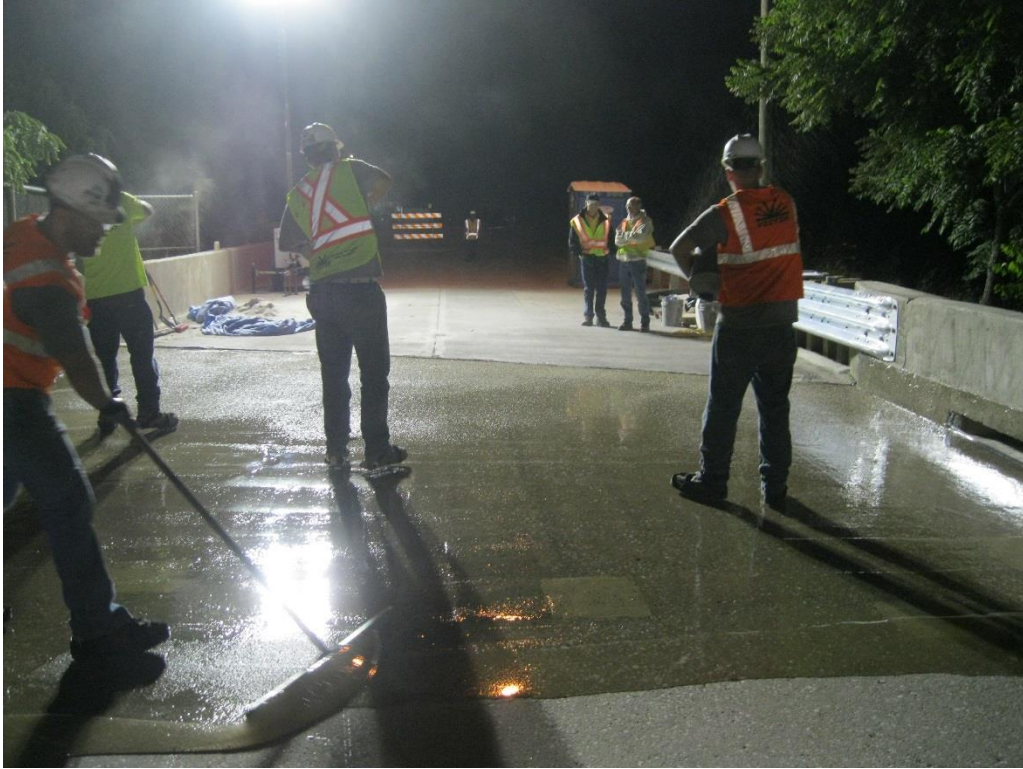
Figure 28. Casting flint chips on Johnson County bridge deck
