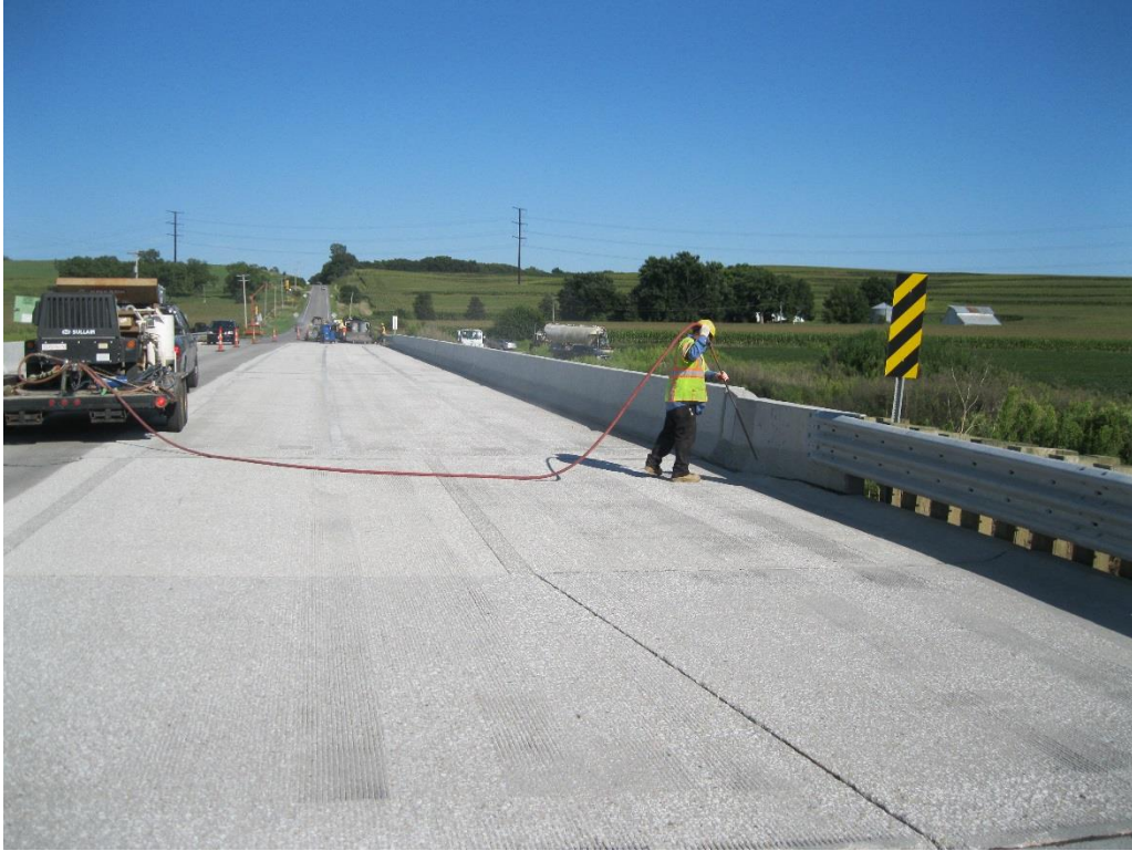
Figure 39. Keg Creek surface preparation
