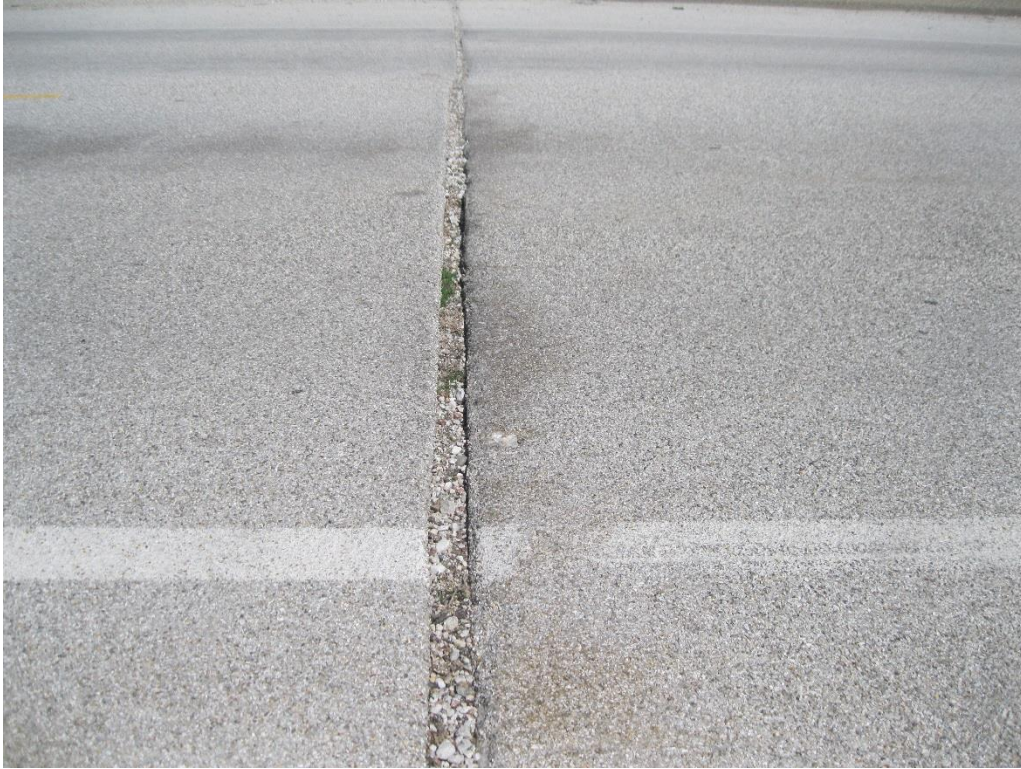
Figure 78. Keg Creek scuffing at bridge entrance
