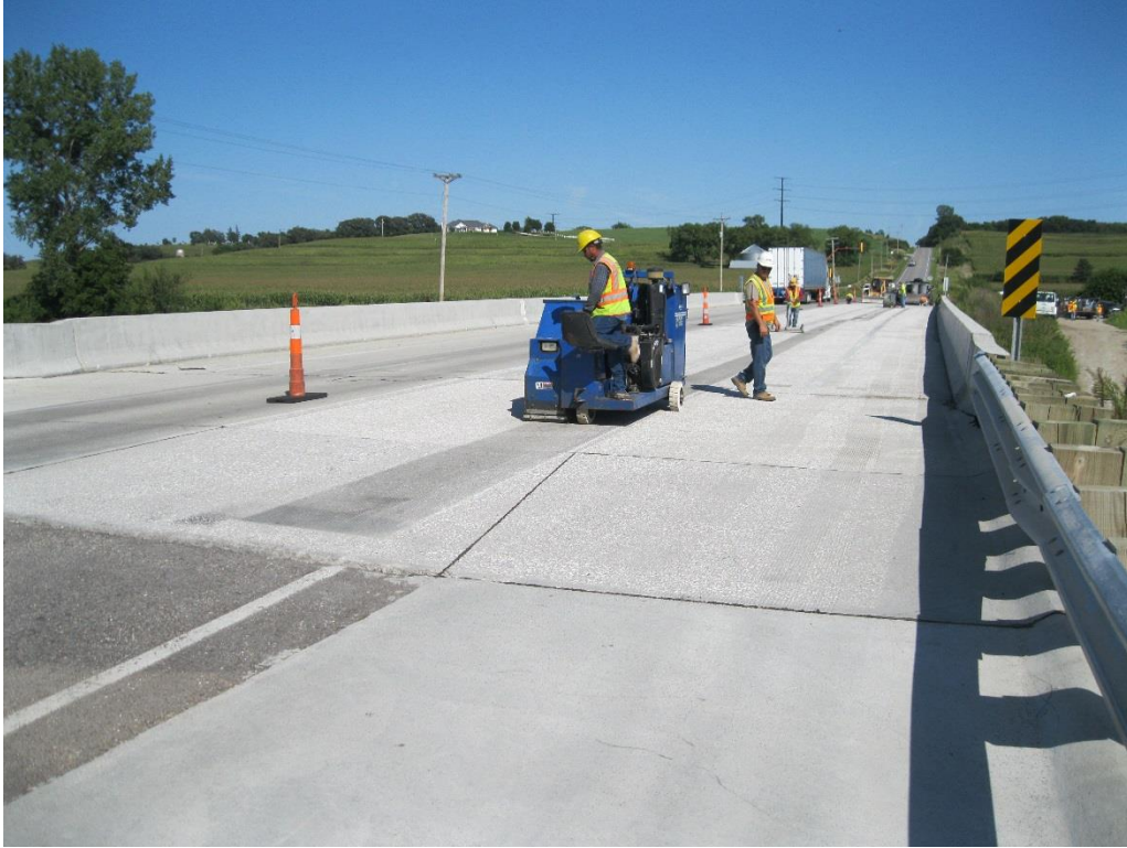
Figure 38. Keg Creek bridge deck shot blasting
