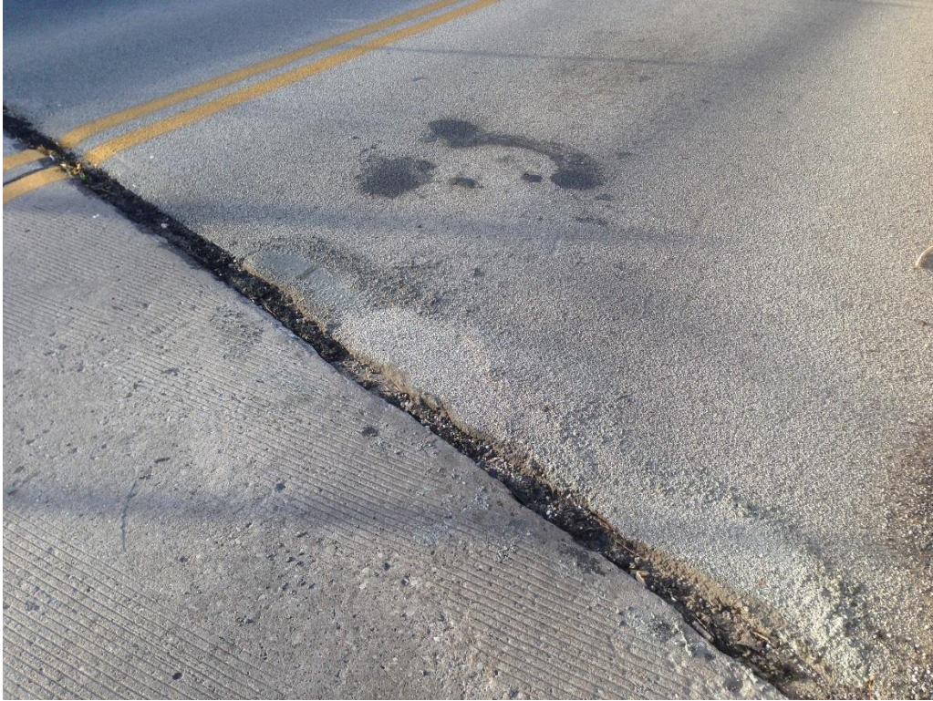
Figure 53. Johnson County epoxy polymer repair at south end of bridge
