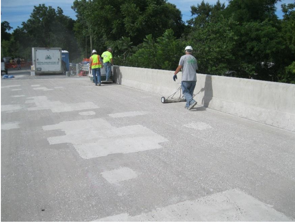
Figure 19. Completed deck repairs on Johnson County bridge
