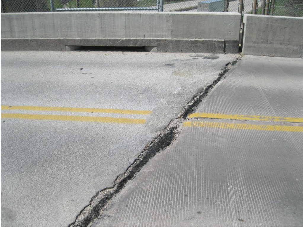
Figure 58. Johnson County epoxy polymer repair at north end of bridge (1 of 2)
