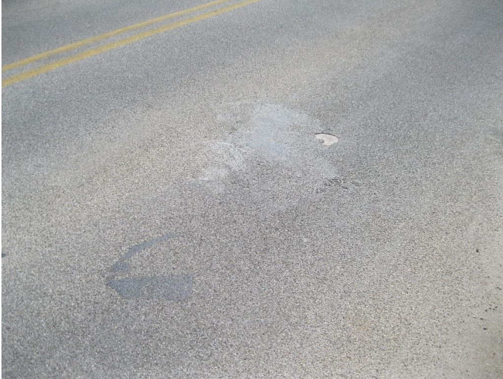
Figure 60. Johnson County delamination in southbound lane
