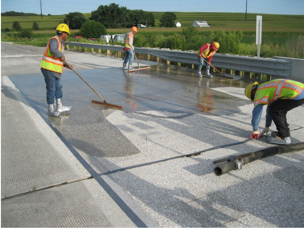
Figure 43. Spreading the polymer on the Keg Creek deck
