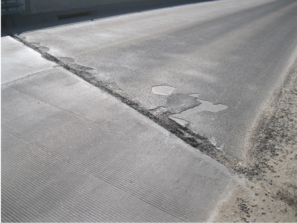
Figure 48. Johnson County delamination at north end of bridge (1 of 2)
