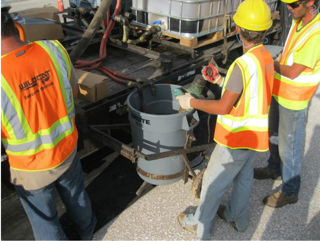
Figure 42. Keg Creek polymer mixing
