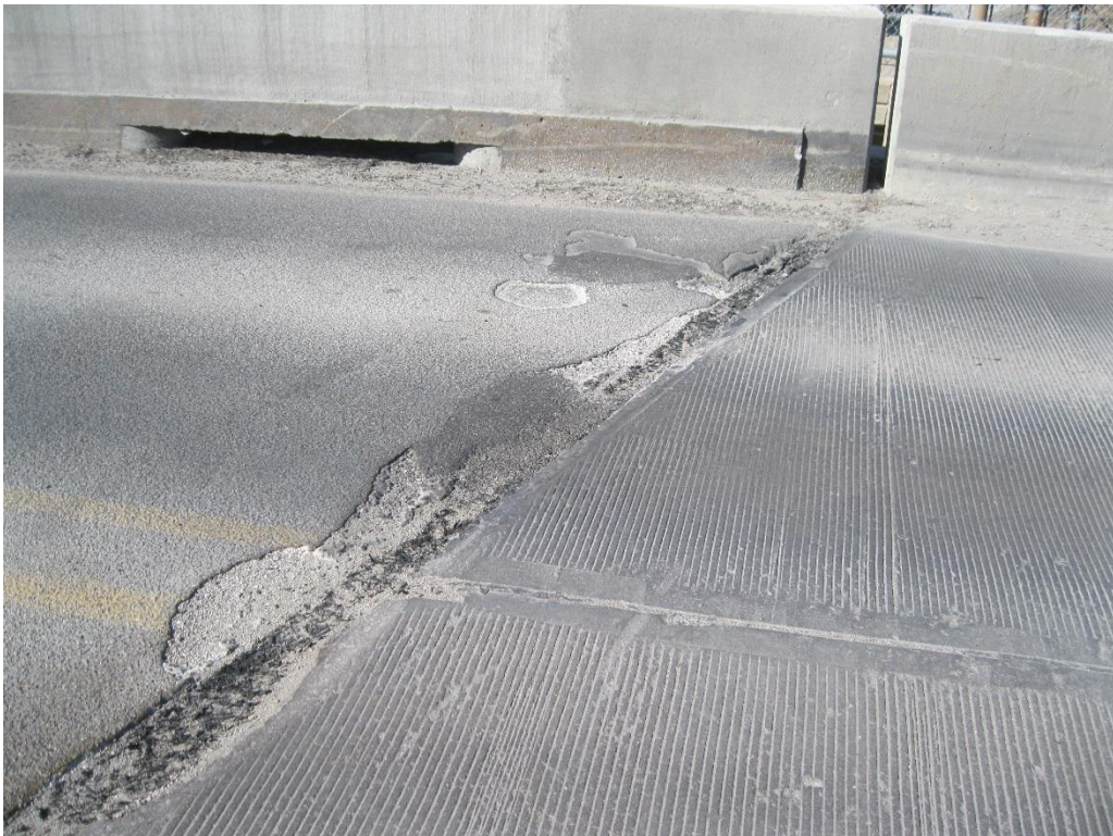
Figure 49. Johnson County delamination at north end of bridge (2 of 2)
