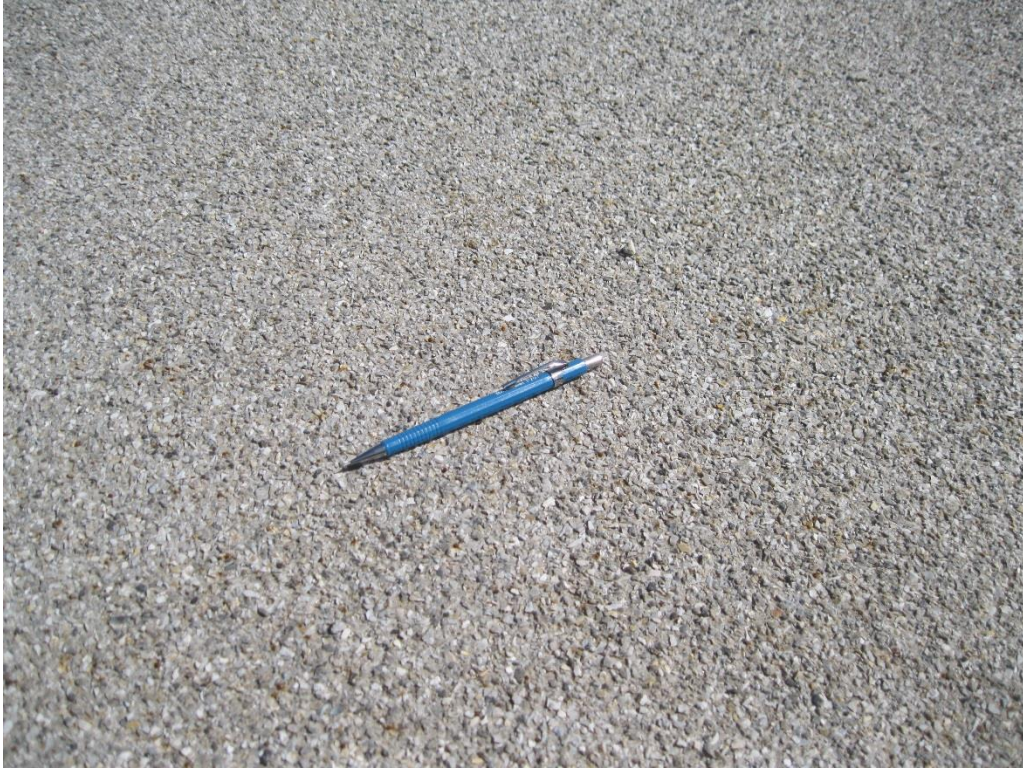
Figure 80. Keg Creek surface roughness where wheel line smoothing
