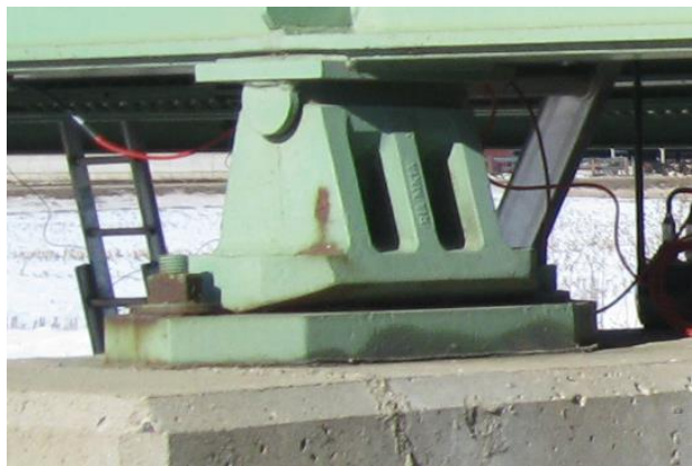
b. Pier bearing
