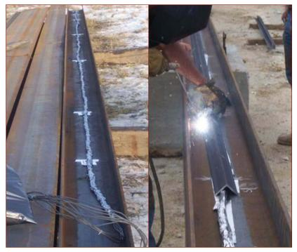
Pile instrumentation (left) and its protection (right)
