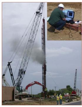
Pile installation with restrikes and PDA (inset)
