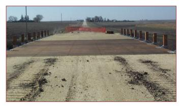
Bridge after plywood and guardrail posts installed
