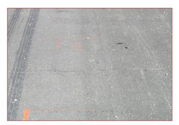
Transverse cracking on Span 1 (with plywood) one year post construction; visible cracking evident at the transverse plywood joints as well as at the panel joints
