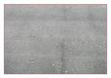
Transverse cracking on Span 1 (with plywood) two months post construction
