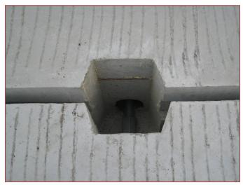
Tie rod block outs in final precast beams for tightening the interior tie rods once bridge components are in place on site
