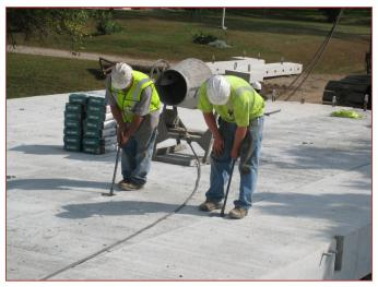
Tightening transverse tie rods before filling block outs with epoxy grout
