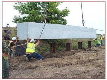
Installing west abutment cap onto pilings before cutting off the lift loops and filling CMP voids with concrete
