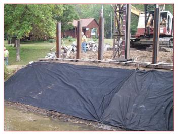
Driving piles with close attention to locations and tolerances using templates to position the five piles correctly
