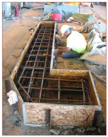
Construction of formwork to precast four back wingwalls, with this being the first ABC project in Iowa to use them
