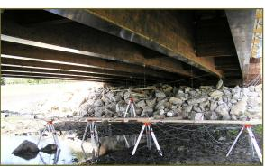
Completed FRP reinforced glulam girder bridge with condition monitoring sensors attached.
