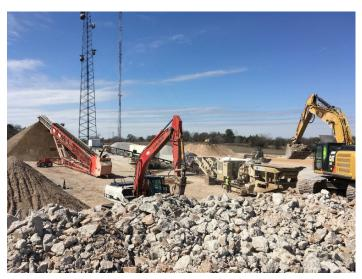
Figure 3. Crushing and sizing of source concrete at on-site stationary plant (photo courtesy of Gary Fick, Trinity Construction Management)
