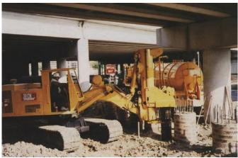
A.H. Beck Foundation Company Figure 2-5. Shaft drilling in low headroom
