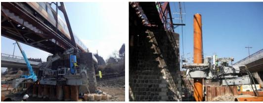
Takuma and Sakai 2018 Figure 3-17. Pile driving using Gyropress method under the bridge
