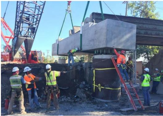
Kang et al. 2017 Figure 3-8. Pre-cast pier cap installation
