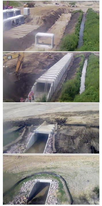
Ida County concrete box culvert construction and earthwork progress July 22, 2016 through November 7, 2016
