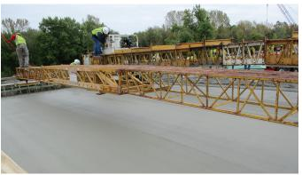
Concrete deck placement in Iowa like that observed and studied for construction factors as part of this study
