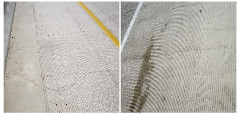
Early-age transverse deck cracks on two Iowa bridges
