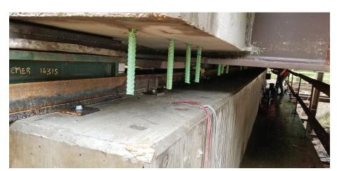
Closure joint between super- and sub-structure during the construction of a multispan bridge using SIBC on IA 1 over Old Man's Creek southwest of Iowa City
