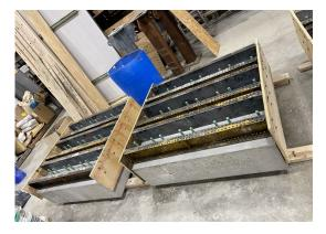
Building the formwork to cast the filling
