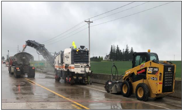
(a) Overview of milling process
