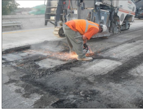
Figure 2.10. Reinforcing steel cut by the milling machine being removed by powered hand saw
