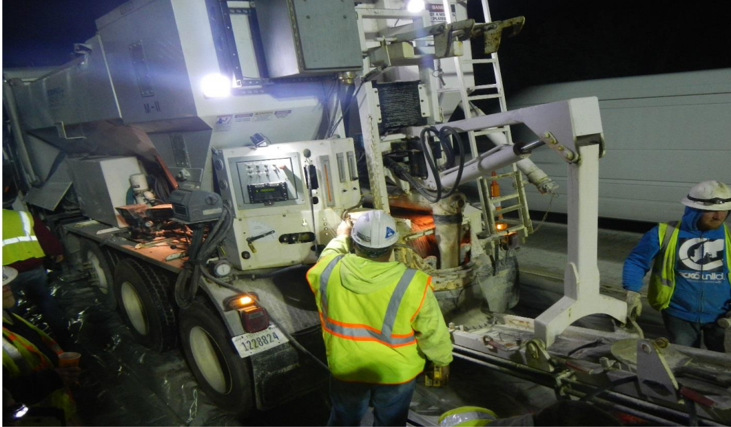
Figure 2.1. Special truck used to mix/discharge LMC
