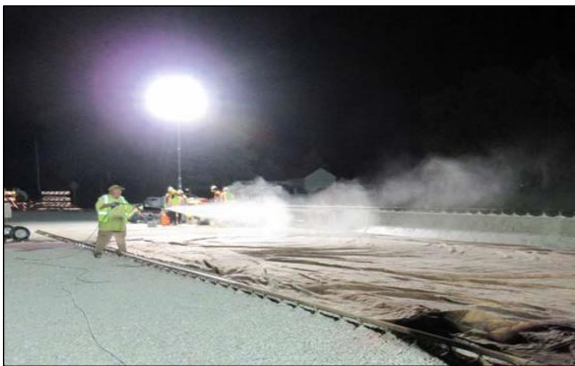
(c) Fogging over the wet burlap cover
