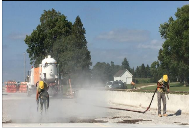
(a) Overview of sand-blasting operation
