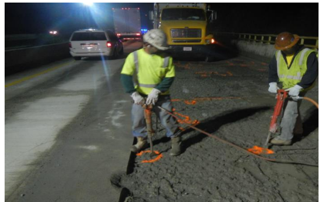
(f) Jackhammering to remove unsound or delaminated concrete detected by the chain drag method after hydro-blasting; resulting debris collected by vacuum truck
