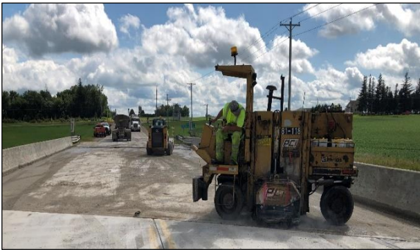
(c) Micro milling at the edges
