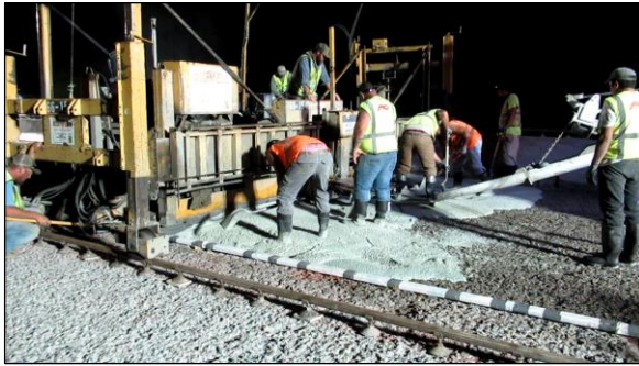
(a) Overview of the overlay casting operation
