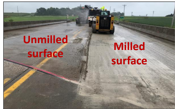
(b) Milled and unmilled surfaces
