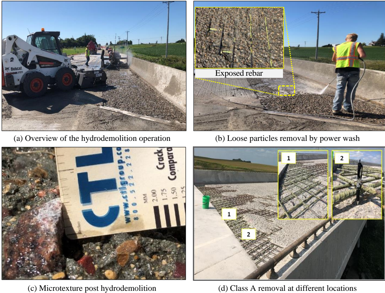
Figure 3.7. Hydrodemolition operation
