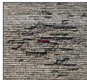
(d) Typical spalled and abraded areas on the overlay concrete
