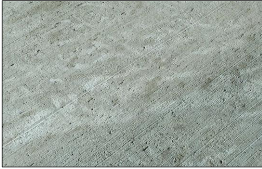
(a) Overlay surface after wet burlap removal
