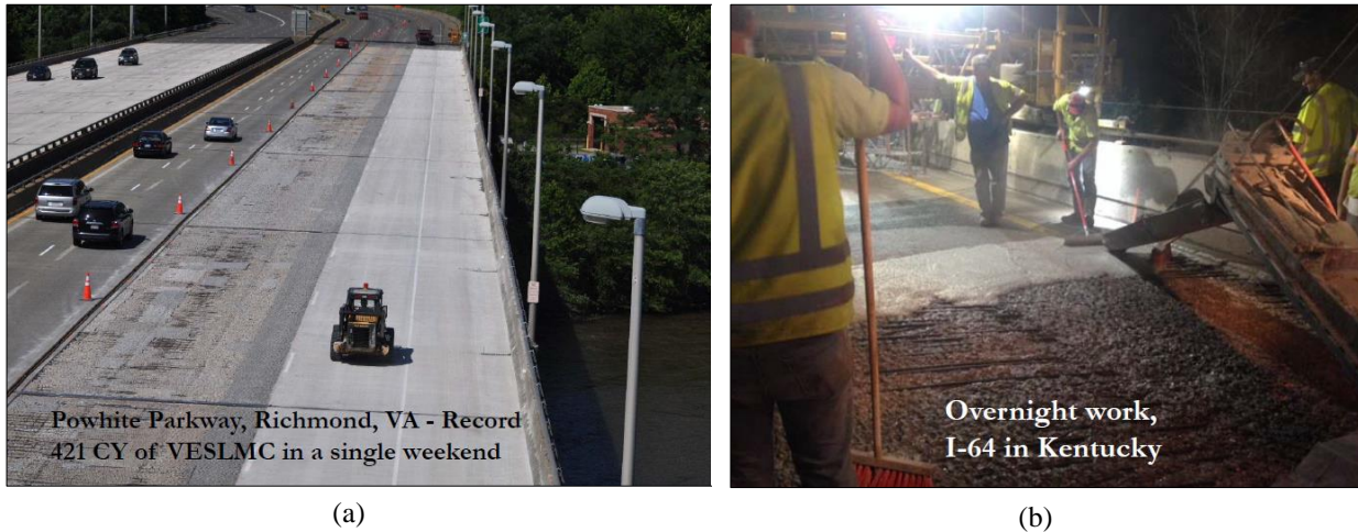
Figure 2.6. LMC-VE overlay construction (a) on a weekend (by VDOT) and (b) overnight (by KYTC)
