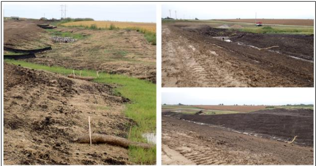
Figure 6. Erosion and sediment control devices at the Oskaloosa site, including wattles
