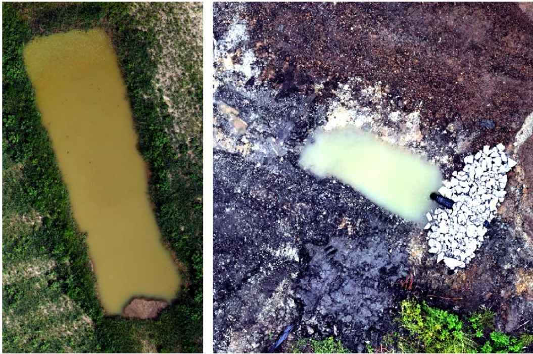
Figure 31. 2D orthophotos showing stormwater basins from Mediapolis Site 1
